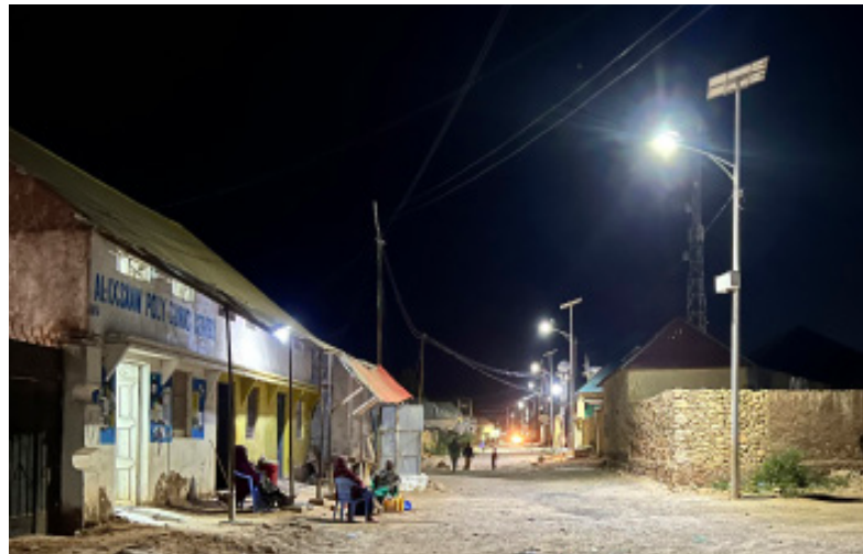
Rehabilitated solar lights in Galkayo
